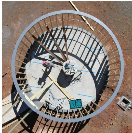
Construction of the ATLAS telescope in Sutherland.
